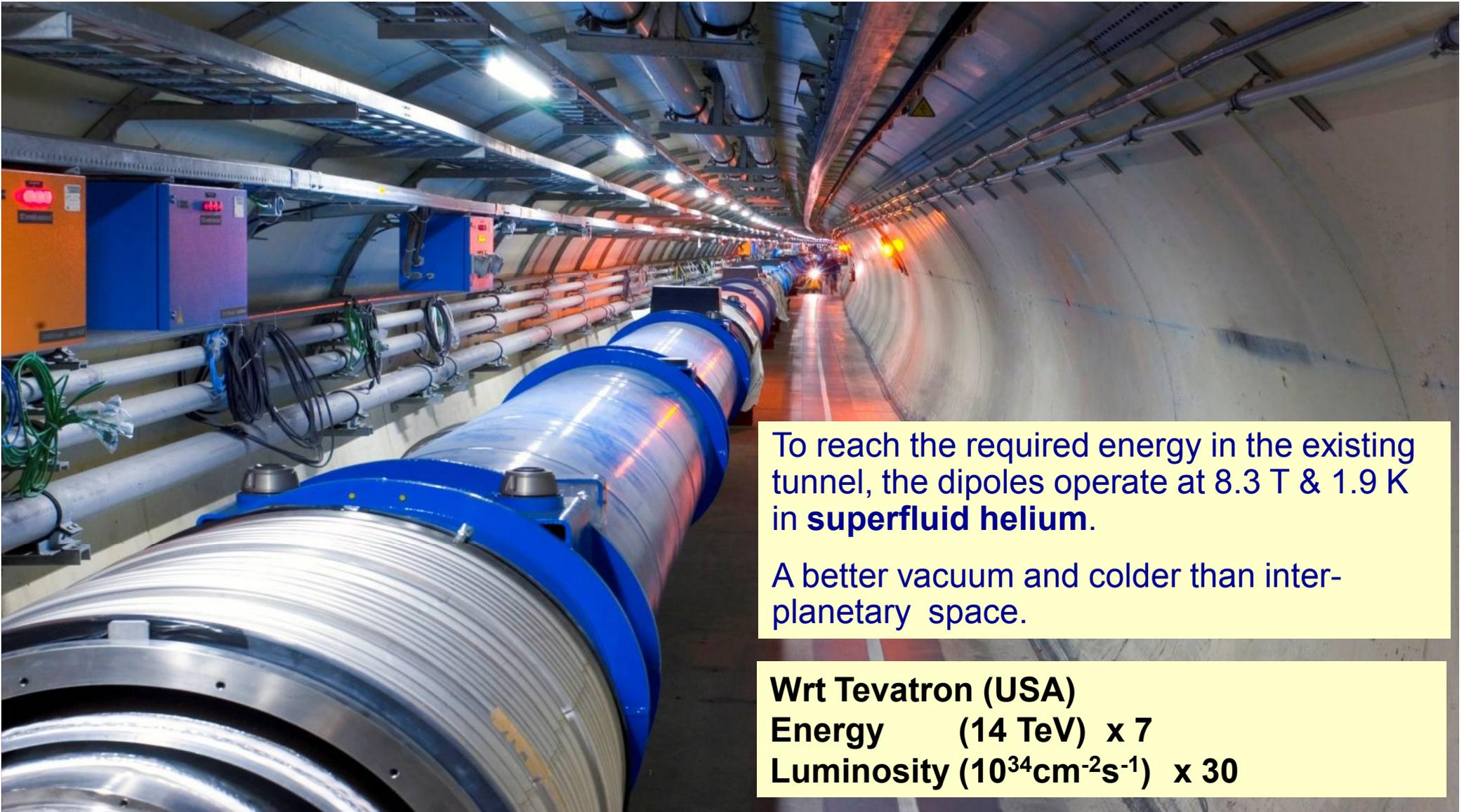
To reach the required energy in the existing tunnel, the dipoles operate at 8.3 T & 1.9 K in **superfluid helium**.
