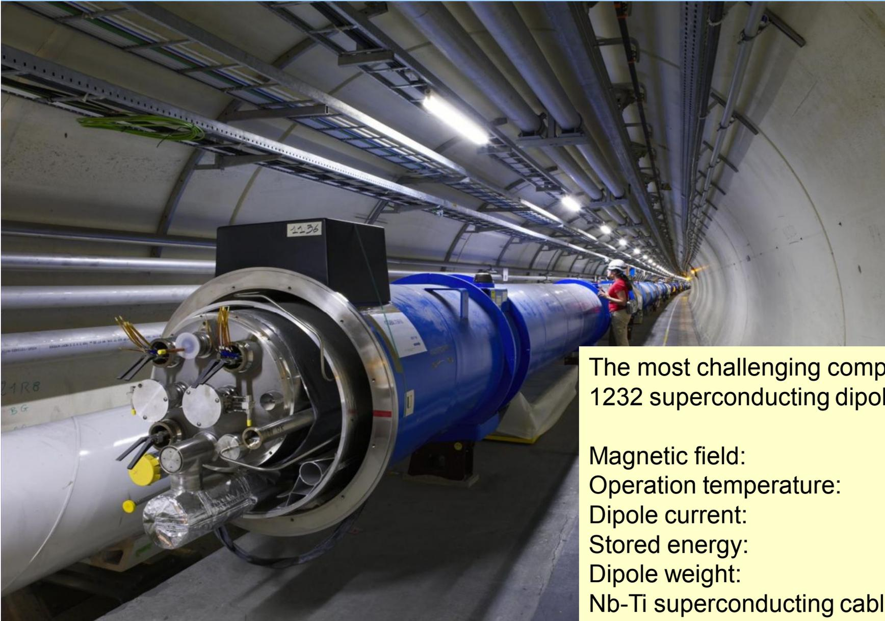
The most challenging components are the 1232 superconducting dipole magnets
